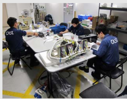
Mechanics performing wiring mod 維修員正在進行線路改裝
